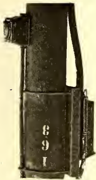
CONDULET ATTACHED TO TROLLEY POLE
